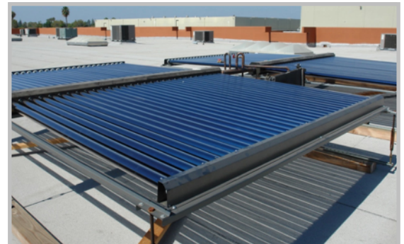
Figure 1. Evacuated tube solar thermal collectors provide heat for the distillation process.
