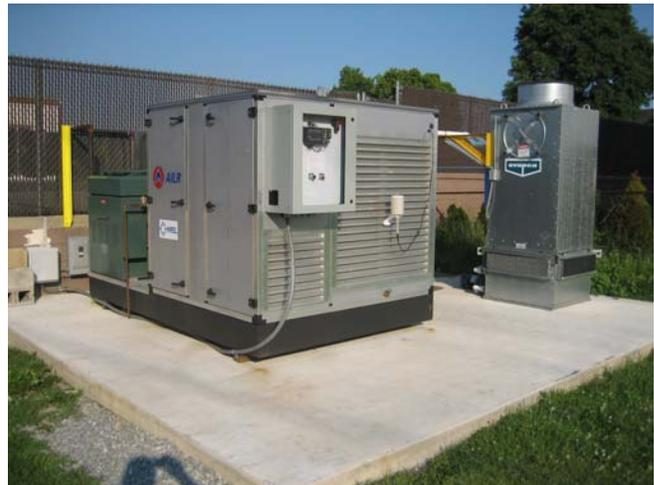
Figure 2 – LDAC Installed as DOAS
